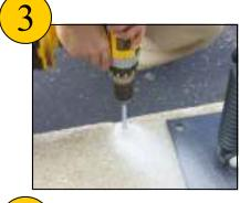
• Use high speed power drill with 1/2" masonry bit and core drill each hole 5" in depth.
