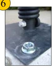
• Tighten concrete wedge bolts until head securely holds base plate to surface.
