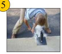
• Using socket wrench with 3/4" drive, thread all four concrete wedge bolts into core drilled holes.
