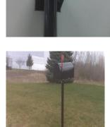
5.) Place mailbox on the post, fitting the Cap over the post. Use provided self tapping screws to attach both components.
