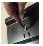
3.) Place washer over the center hole in the post cap and screw in the Cap Bolt using the provided Hex Key (Allen Wrench).
