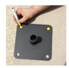
Mark the four base holes to be drilled.
