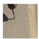
Use high speed power drill with 1/2" masonry bit and core drill each hole 5" in
