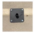
Tighten concrete bolts until head securely holds base plate to surface.
