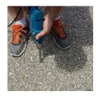
Use high speed power drill with 3/4" masonry bit and core drill each hole 6" in depth.
