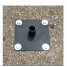
Tighten hex screw until head securely holds base plate in place
